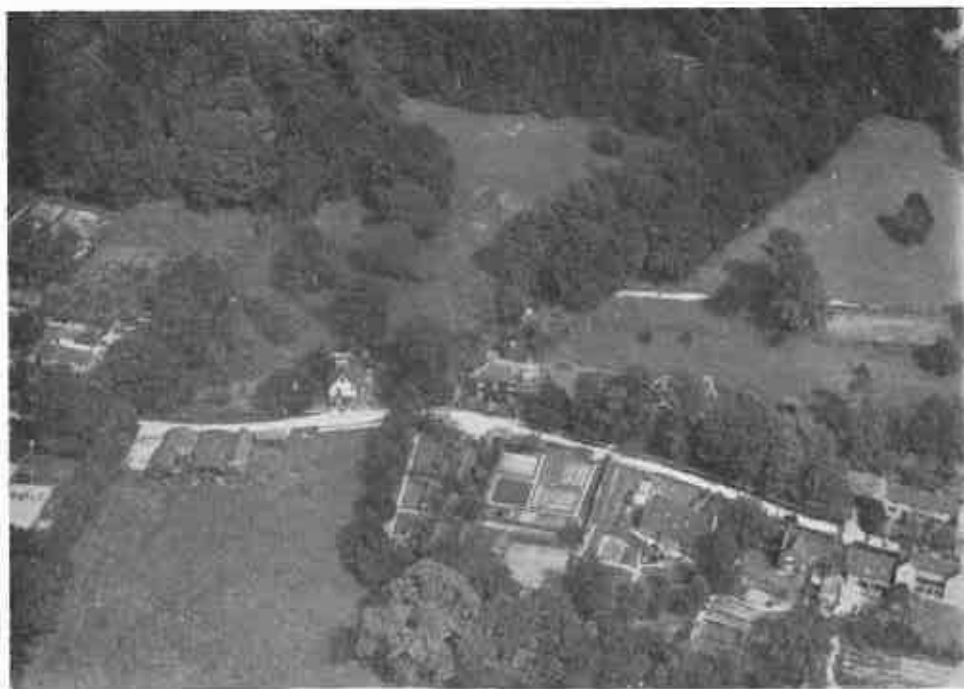
Aerial View from the West
